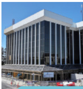
New City Hall Construction
