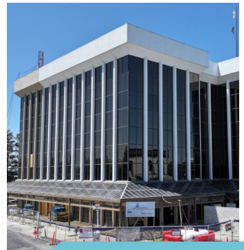
New City Hall Construction
