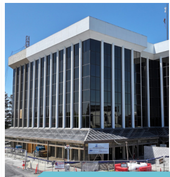
New City Hall Construction
